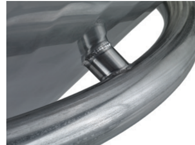
FCX Stainless Steel Weld Detail
